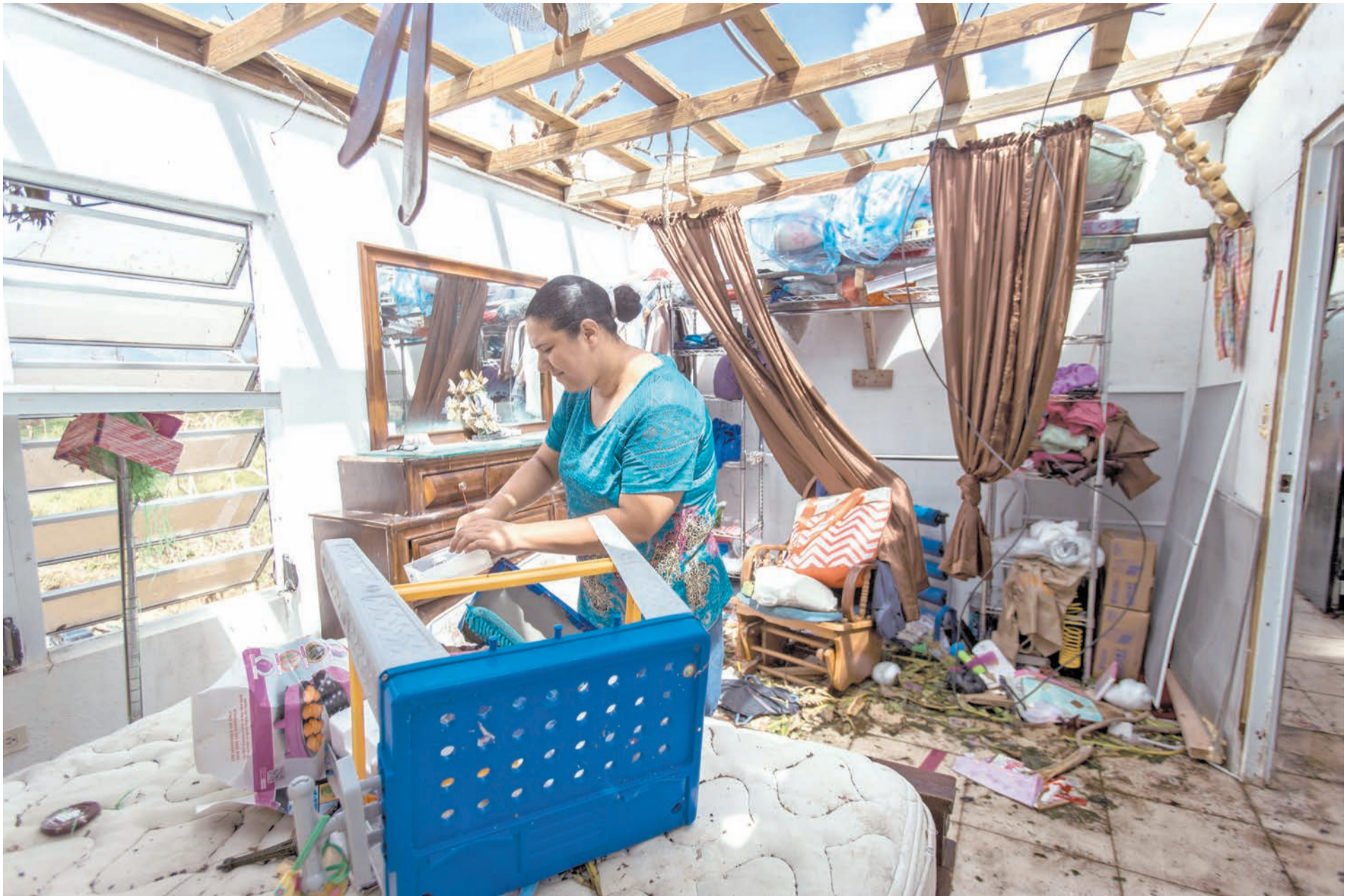
Meryanne Aldea lost everything at her house in Juncos when the winds of Hurricane Maria ripped away the roof. The Puerto Rico town remains largely isolated from the rest of the island - and the world. MUST CREDIT: Photo for The Washington Post by Dennis M. Rivera Pichardo
